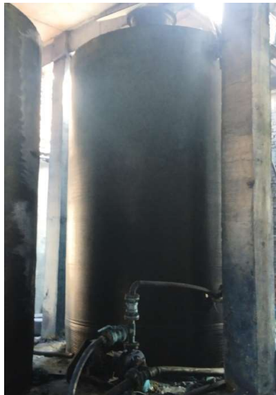
Spent Acid Storage Tank
